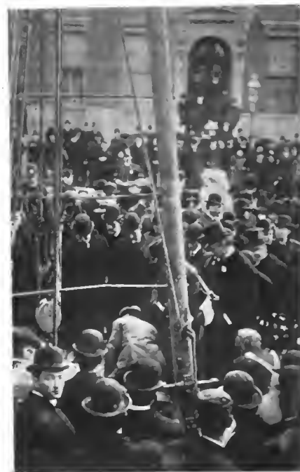
THE LAYING OF THE STONE.
